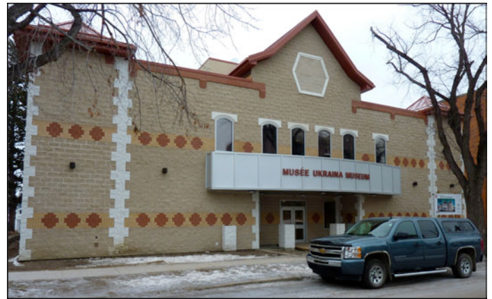
Dec. 15, 2011. Construction of Museum nears completion.
