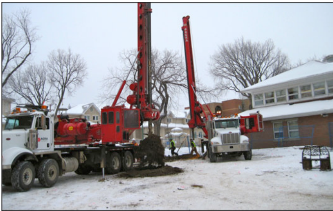
Construction begins Dec. 20, 2010
